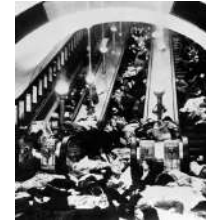
Underground Station Shelters
